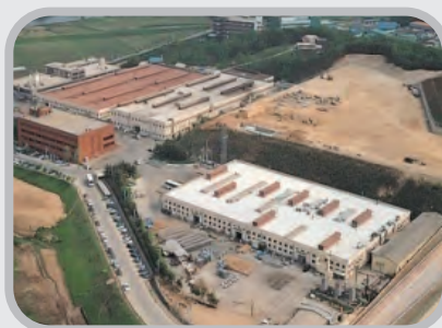
• Hwaseong 1 st Plant
