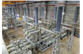
362kV GIS Outdoor substation
