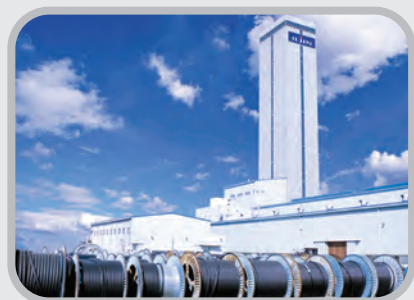
• Hwaseong 2 nd Plant
