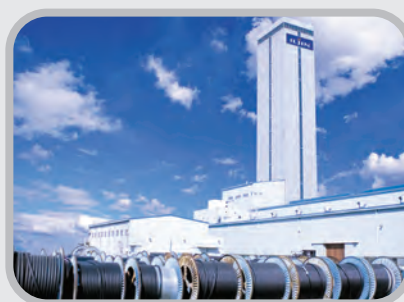
• Hwaseong 2 nd Plant
