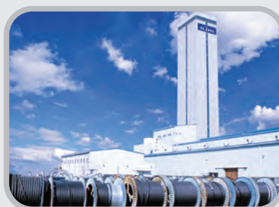
• Hwaseong 2 nd Plant
