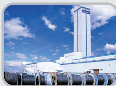
• Hwaseong 2 nd Plant
