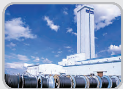
• Hwaseong 2 nd Plant
