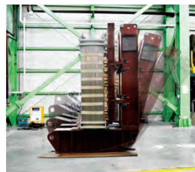
· ERECTION OF CORE ASSEMBLY
