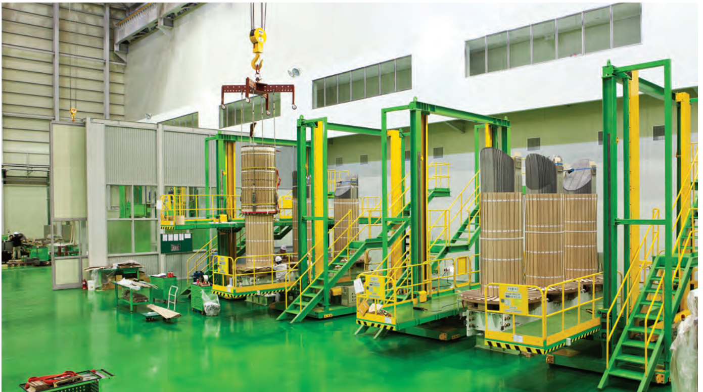
· CORE AND COIL ASSEMBLY SHOP
