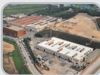
• Hwaseong 1 st Plant
