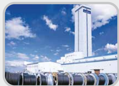
• Hwaseong 2 nd Plant
