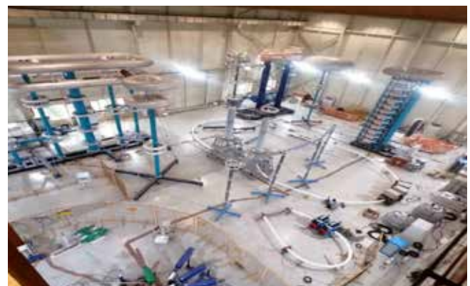
[ ±320kV VSC type XLPE cable system Type test loop ]
