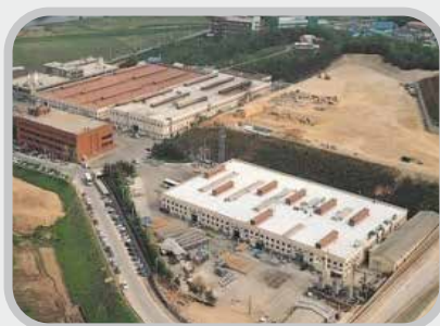
• Hwaseong 1 st Plant
