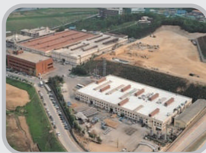
• Hwaseong 1 st Plant
